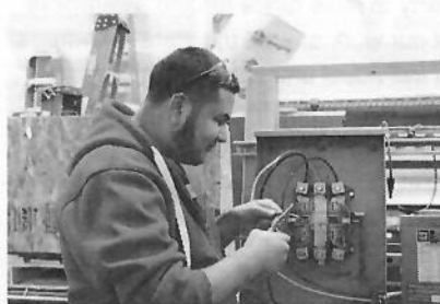
A trainee from Mile High Youth Corps learns about solar wiring in Denver.
