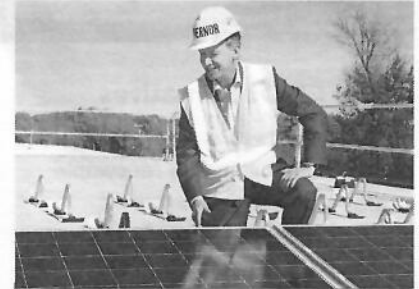
Governor Hickenlooper on the roof with GRID in Fort Collins.
