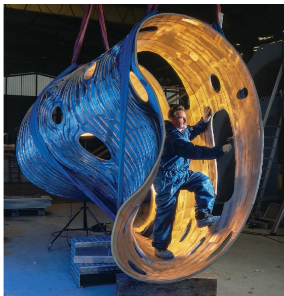
Wendelstein 7-X's bizarrely shaped components must be put together with millimeter precision. All welding was computer controlled and monitored with laser scanners.
