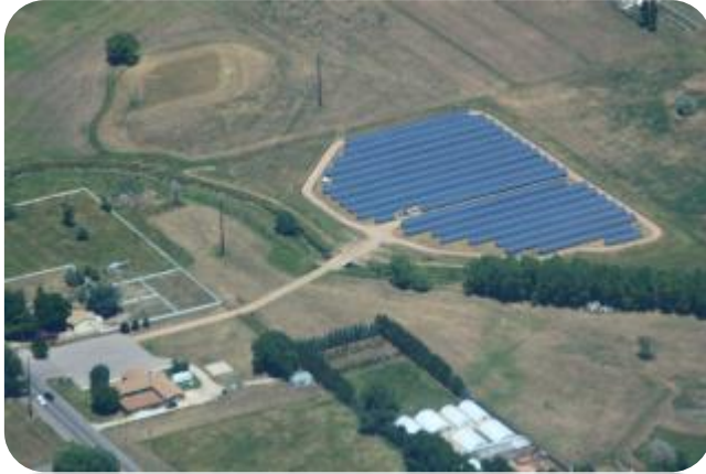
LaPorte Solar Farm 1 MW
